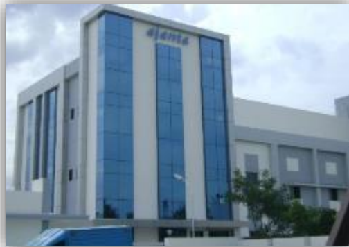
API Plant - Waluj
