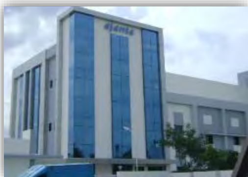
API Plant - Waluj
